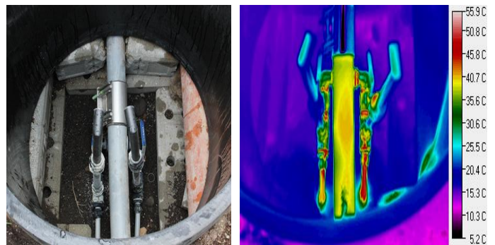
Figure 7: Overhead view of the NLFI test bed connections detail photo left, infrared image right. Note the plastic air vent pipes on the bottom of the left photo correspond with the light blue pipes in the right photo.
