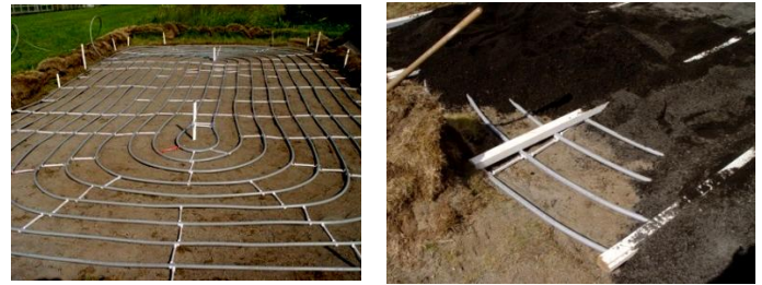
Figure 2: Hveragerdi spiral piping layout (left), sand over layer construction detail (right).
