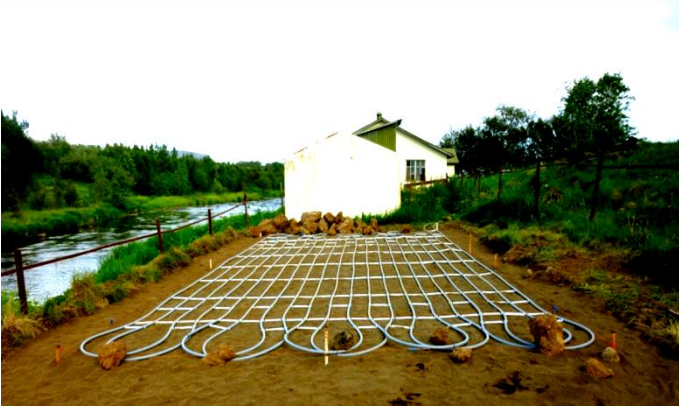
Figure 8: The pipe layout for the test bed at Varmá.
