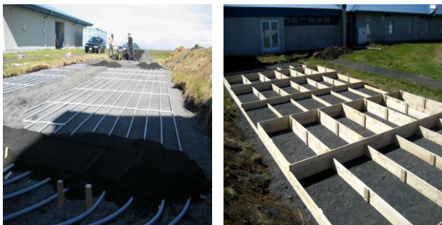
Figure 4: The construction of the Keilir garden.
