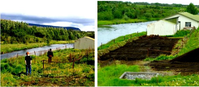
Figure 9: Left, before garden construction, right, after garden construction. The rectangular concrete and stone cooling pit for the waste hot water is visible in foreground of the right image.
